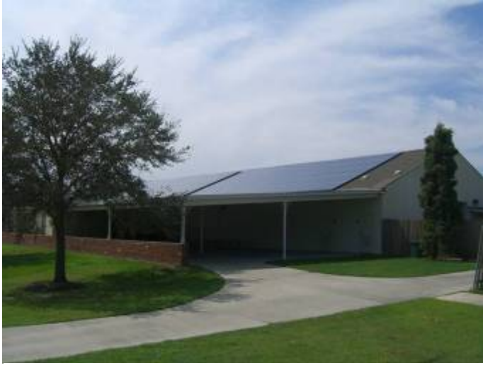
Solar cells on the cart barn. Courtesy of Gulf South Solar
