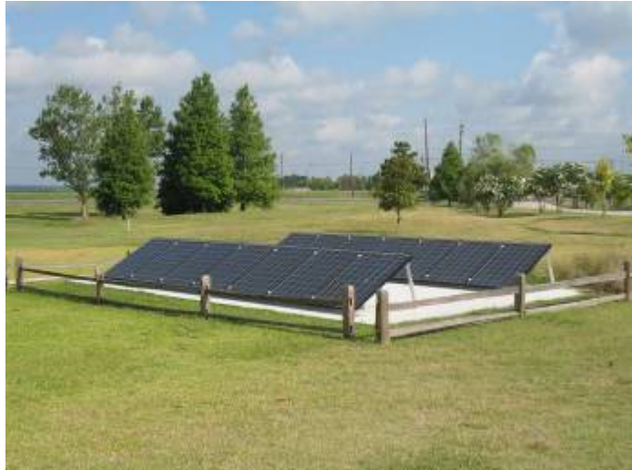
Second solar system for groundwater pump. Courtesy of Gulf South Solar
